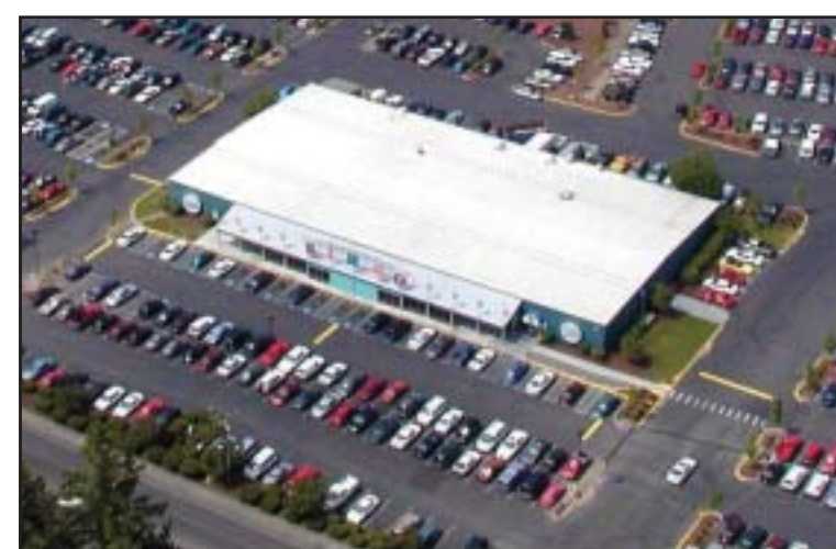
Aerial Shot of the old bingo hall shortly before it was demolished.
